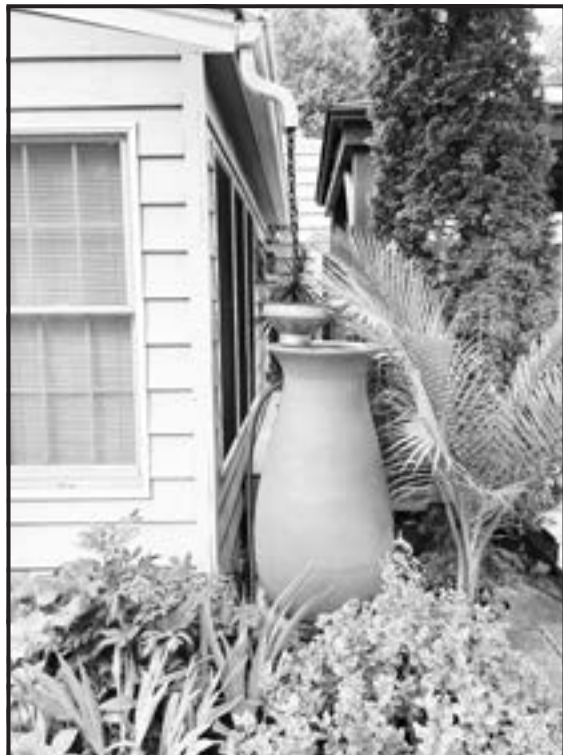
Rain barrels can help manage the water on your property and provide water to use in your gardens.
