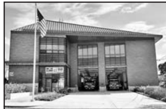
Brand new firehouse which just opened a few weeks back. (Courtesy photo by BFD)
